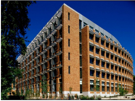
Computer Science & Engineering Building at University of Washington
